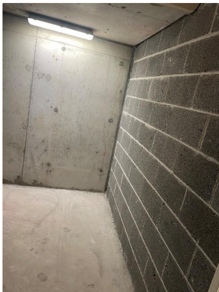
Figure 3: Fire egress stair not containing fire hydrant.
