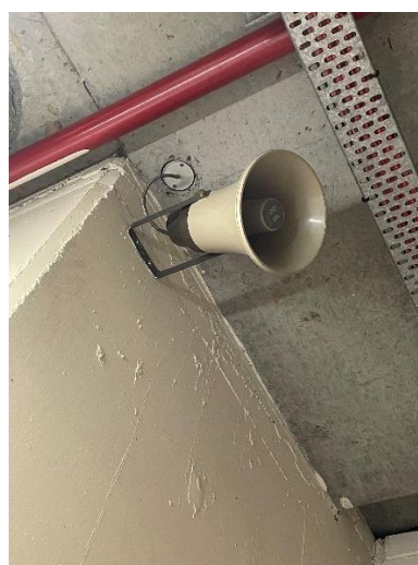
Figure 19: EWIS horn speakers and strobe lights
